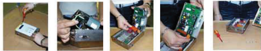
Fig. 28: Replacing a controller
